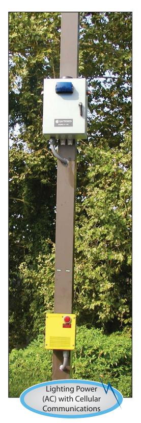
**Solution**: GAI-TRONICS offers a pole-mounted solution similar to our tower package designed to utilize lighting power that is available only at night. During these hours, the included batteries will charge, providing power during daylight hours when no lighting power is available. This package includes:
